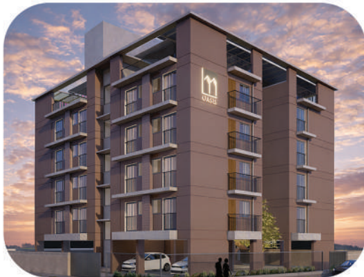
SMS Oasis, Thoppumpady (Ongoing)
