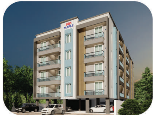
SMS Maple, Edappally (Ongoing)
