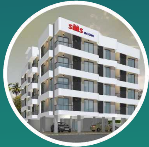
SMS BODHI Edappally (Ongoing)
