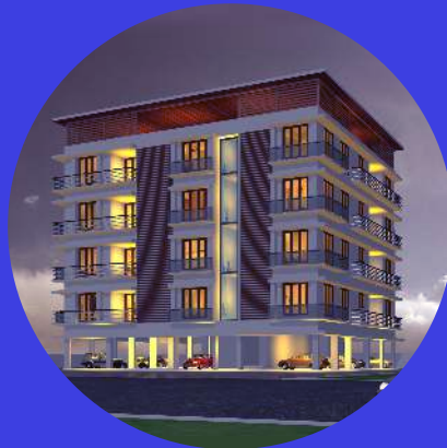
SMS SERENITY II Panampilly Nagar (Completed)
